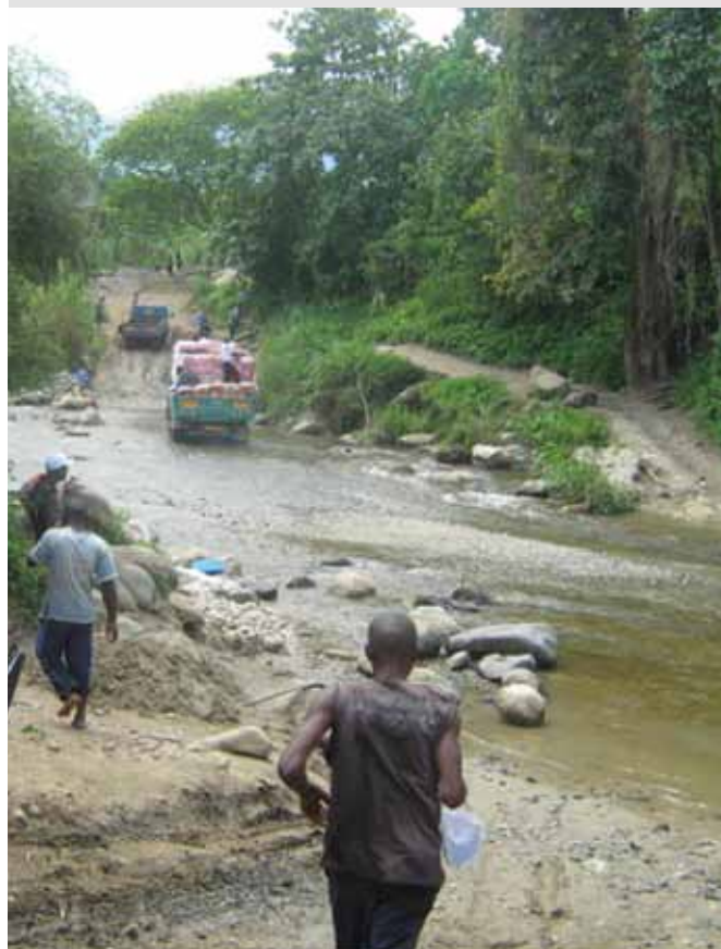
Below: Damaged infrastructure in Bundibugyo
