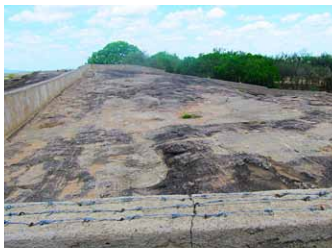
Rainwater harvesting through a rock catchment dam in Kotido, supported by Oxfam GB
